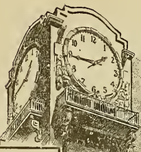
Tower clock wound automatically by one-half horse power motor.
